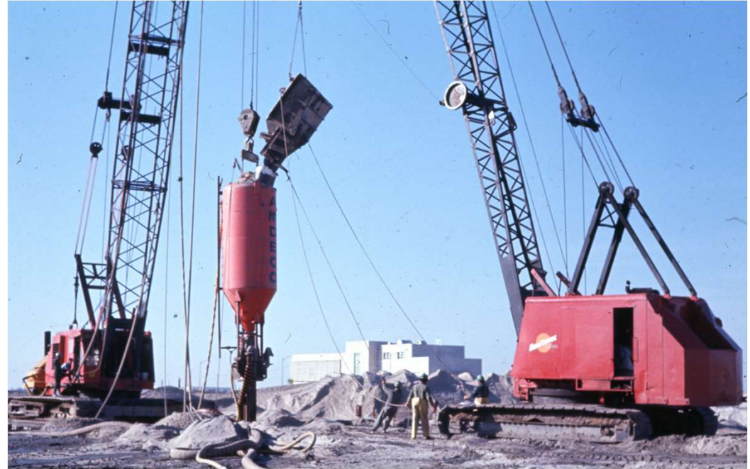
Sand Drain Installation on South Island Expansion – 1970s
