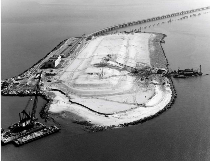
Construction of South Island Expansion with Surcharge – 1970's
