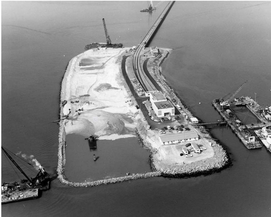
Construction of North Island Expansion with Surcharge – 1970's
