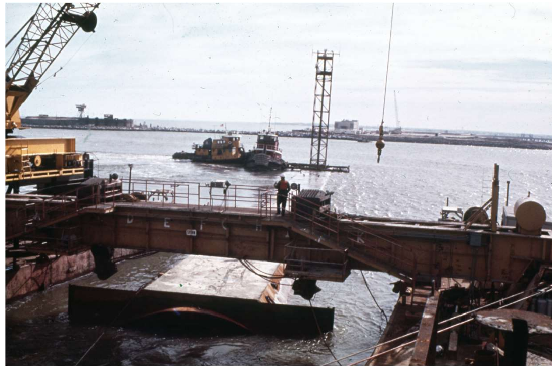
Immersed Tube Tunnel Placement – 1970s
